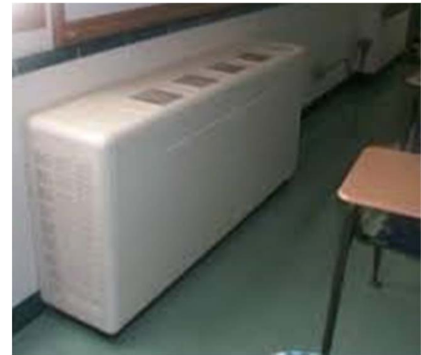
unit ventilator (fan)
