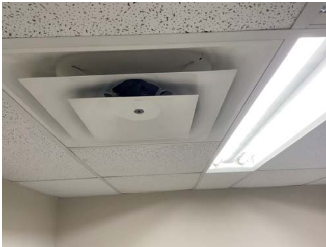
HVAC ceiling diffuser
