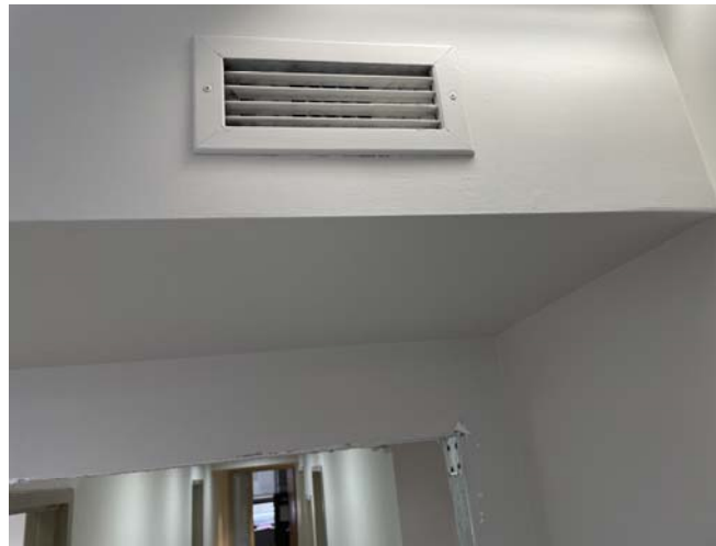
HVAC wall diffuser
